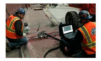
Comply with API and similar fabrication codes using Olympus' complete PA solution for liquified natural gas (LNG) tank inspection. WeldSight™ software increases productivity and provides real-time analysis, compared with RT or UT systems. Inspect the austenitic 9% nickel shell to I625 dissimilar metal welds that are typical of cryogenic storage tanks using our DLA probes.
